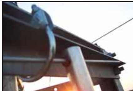
A 9 wavelength 432 yagi is supported temporarily by it's front director element leaving both hands free to do something else.
