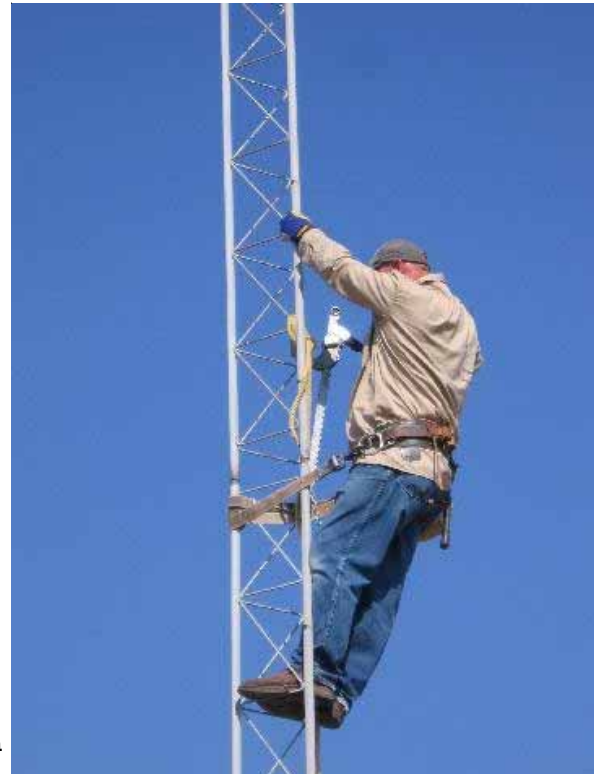
#4 remove tower sections with jack!
